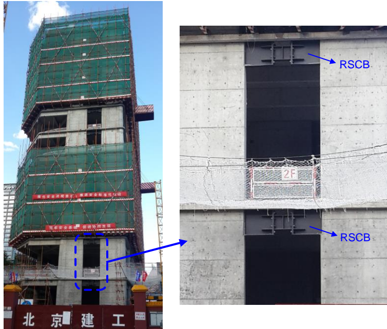
(a) Photograph of prototype building under construction
